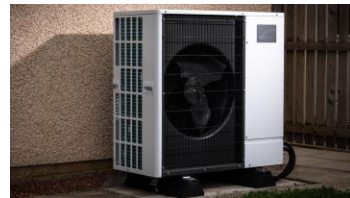
Air to Water Heat Pump
